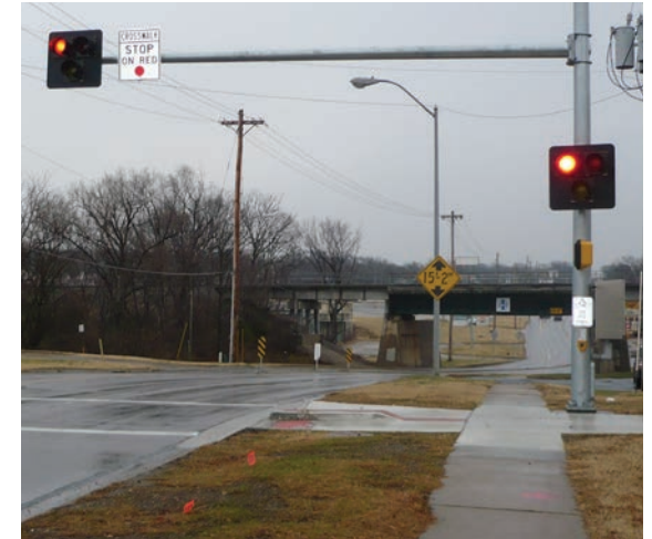
The Hybrid Beacon or HAWK signal. This three-headed pedestrian actuated device is normally dark. When activated by a push button, its single amber light flashes to warn motorists of an impending red signal. The two upper heads then turn red to stop traffic.
