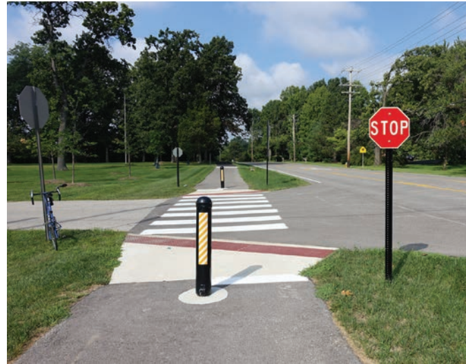
Sidepath with well-marked crossing, Clayton Road in Saint Louis County, MO
