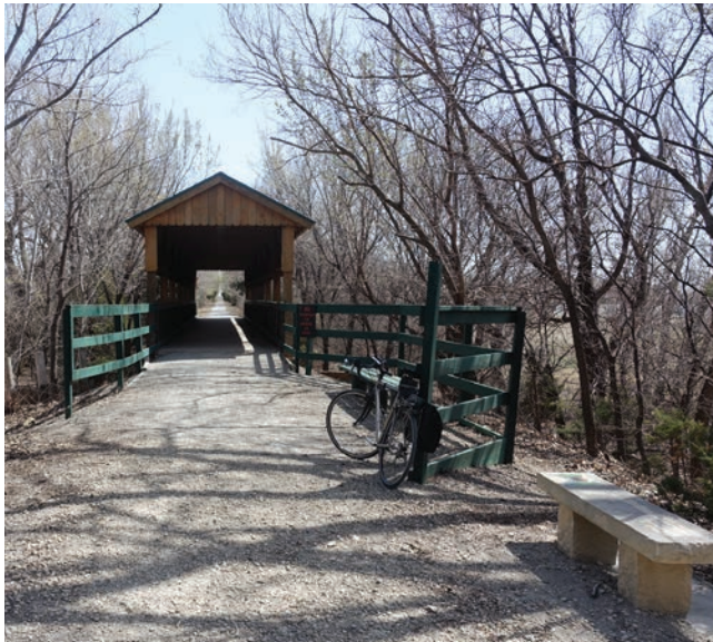
The Prairie Sunset Trail in Garden Plain, Kansas. This trail between the west edge of Wichita and Garden Plain converted a disused rail corridor into a rural shared use path, surfaced with granulated stone. The trail was developed and is operated by the nonprofit Prairie Travelers Inc.
