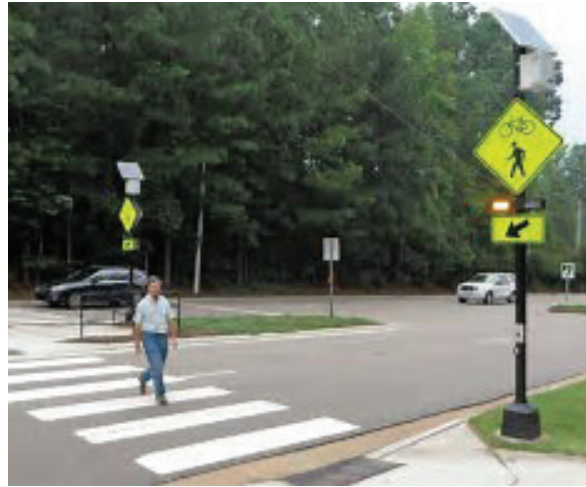
Rapid Rectangular Flashing Beacon (RRFB). This pedestrian activated device has twin, very bright beacons that flash alternatively and very effectively indicate the presence of pedestrians in a crosswalk to motorists. However, they do not include a red signal.
