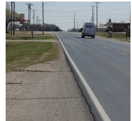
Harry Street Existing Condition
