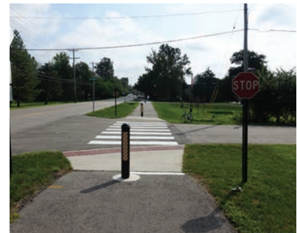
Good sidepath intersection design: Ramp is directly in line with travel path, crosswalk is unobstructed and clearly marked.
