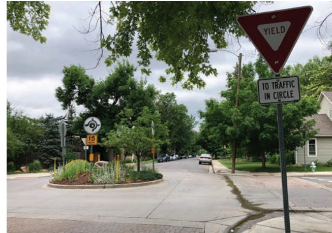
Traffic calmer on a bicycle boulevard in Boulder, CO
