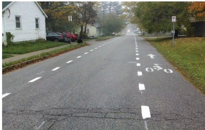
Advisory bike lanes in practice. From top: Used in combination with a defined parking lane; along a narrow rural road (both photo credits: Alta Planning + Design); and in a contrasting pavement color in a downtown setting.
