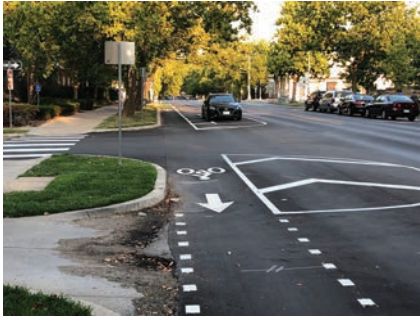
Above: a good intersection design, with painted or raised bump-outs that provide better visibility for a protected bike lane and also benefits pedestrians who are crossing wide streets (Armour Boulevard in Kansas City)
