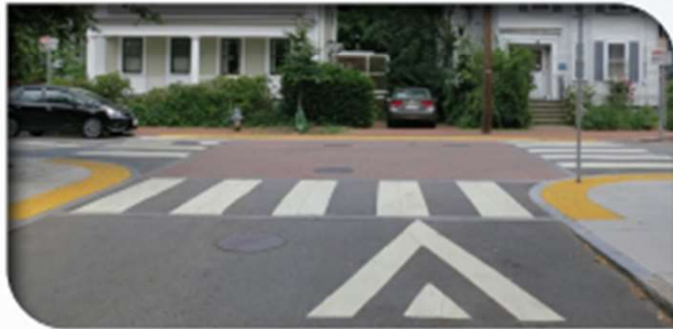
Source: Raised Crosswalk, City of Cambridge, Massachusetts:
