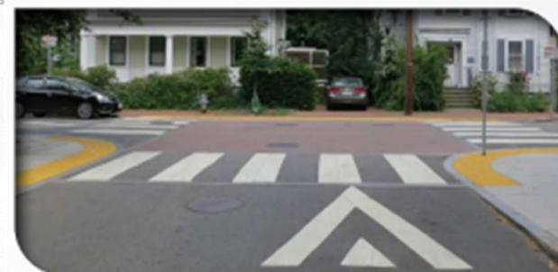
Source: Raised Crosswalk, City of Cambridge, Massachusetts
