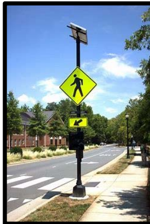
Left: Solar Powered Crosswalk Sign
