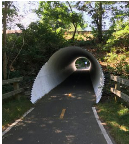
Greenway Railroad Crossing Tunnel
