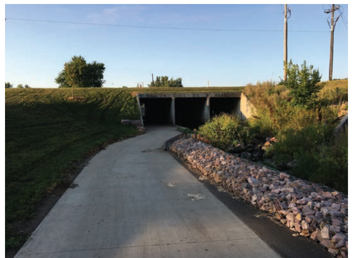
Multi-lane roadway underpass. Sioux falls, SD
