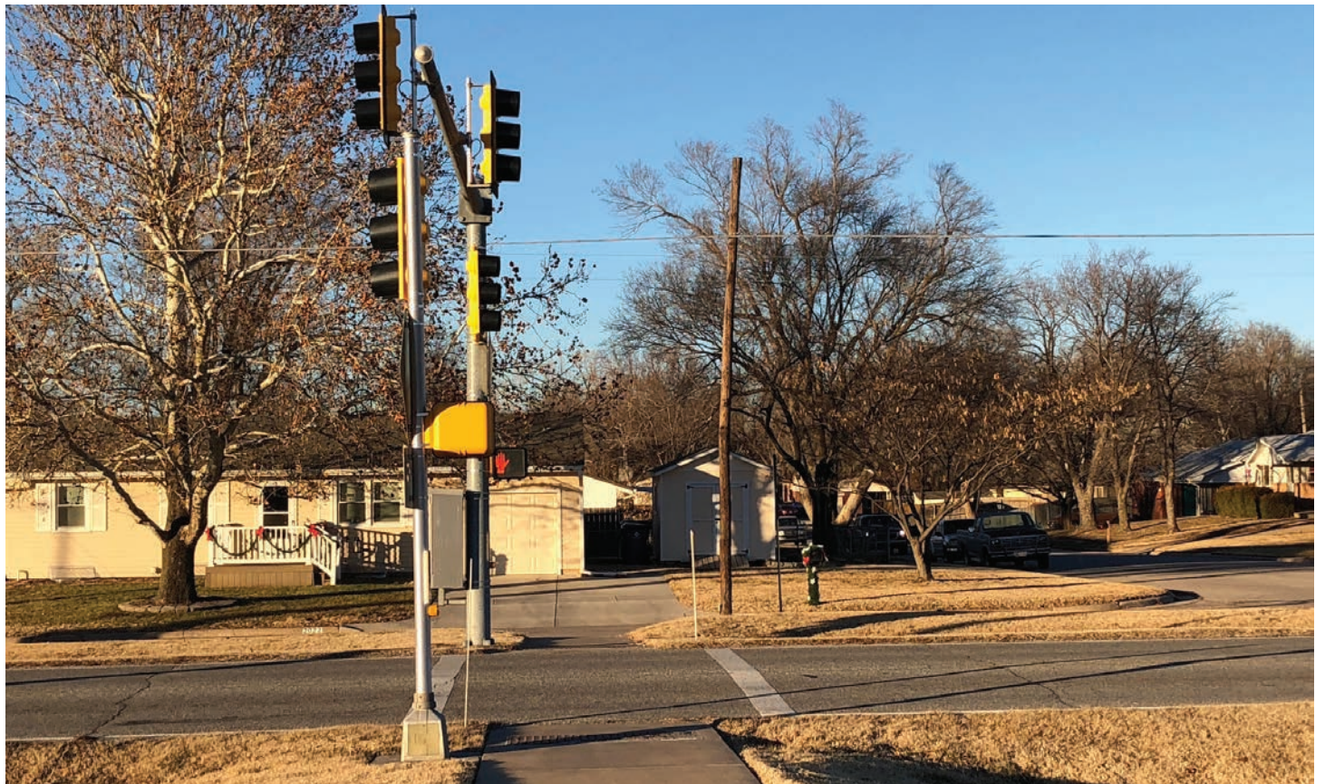
Phase 1A includes upgrading key crosswalk markings to high visibility, reinforcing awareness of pedestrians in the area at both signalized and unsignalized crossings.
