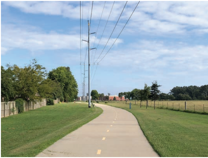
Shared use path along transmission line easement. Razorback Greenway between Fayetteville and Bentonville, AR
