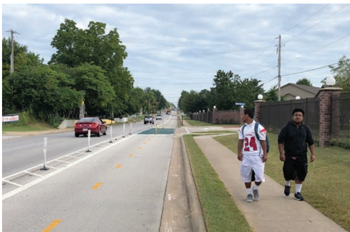
Complete street concept along the Razorback Greenway in Springdale, AR, with sidewalk, protected two-way bike lane, and travel lanes on a major collector corridor
