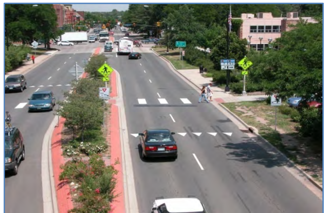
Example of pedestrian refuge islands with pedestrian actuated signals that stop traffic only when a user is present, visible crosswalks, and appropriate signing.
