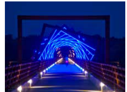
Signature bridges. Top: North Freeway pedestrian bridge, Omaha. Middle two: US 75 bridge concept on Flint Hills Nature Trail near Lyndon, KS; High Trestle Trail near Madrid, IA
