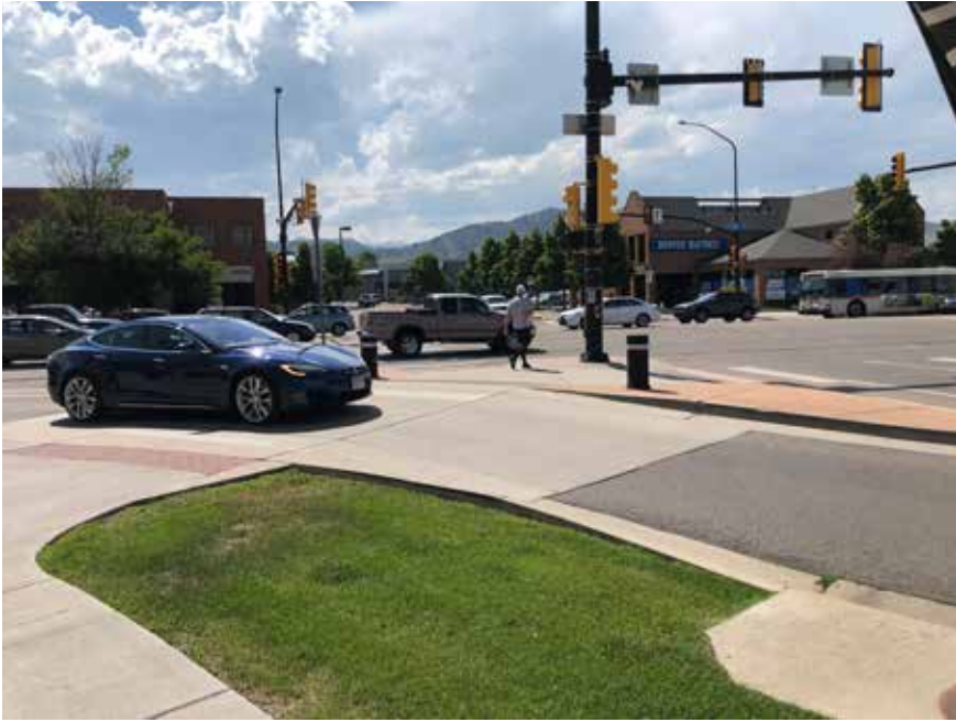
Pedestrian crossings: From left: Right turn bypass provides a generous refuge area between right turning and direct traffic (Boulder); intermediate medians improve comfort of crossing a major arterial (Green Bay)
