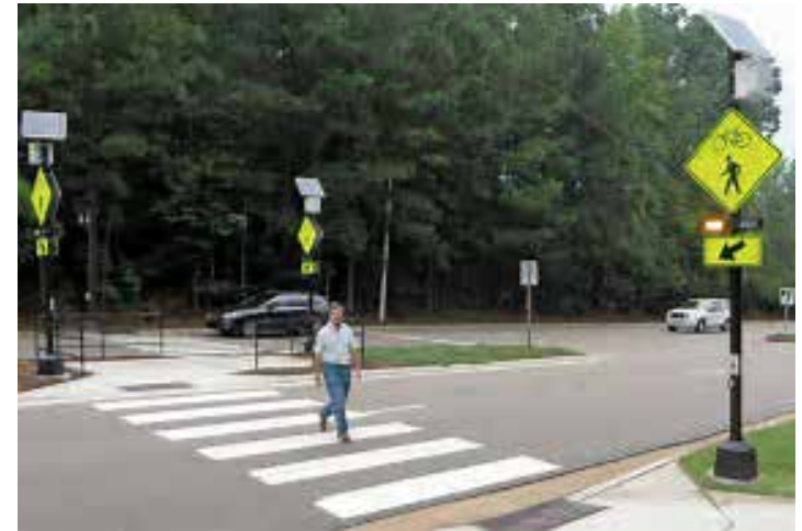
High visibility crosswalk with Rectangular Rapid Flashing Beacon
