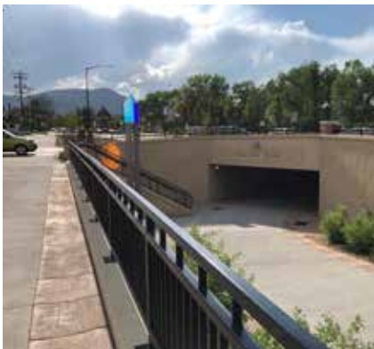
Trail underpass across major arterial, Boulder, CO
