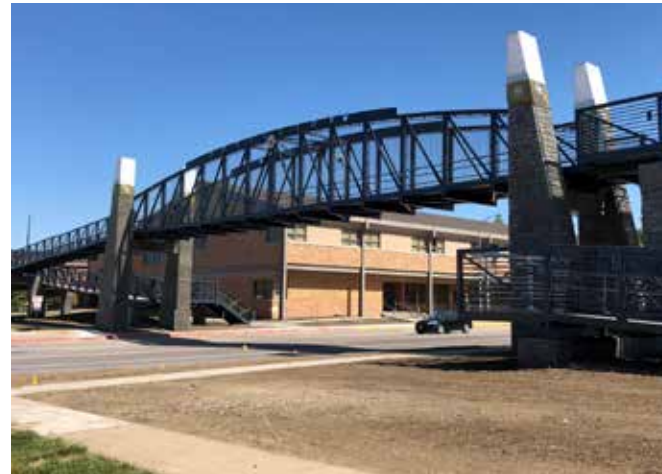
Pedestrian bridge in Papillion, Nebraska. This bridge has a span approximately equivalent to that of Kellogg Avenue at a construction cost (excluding design, testing, and other costs) of about $1.8 million.
