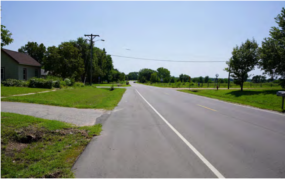
22 / Tracy Avenue's wide shoulder could be converted to an on-street pedestrian lane.
