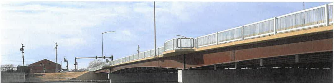
W Lincoln Street Bridge
